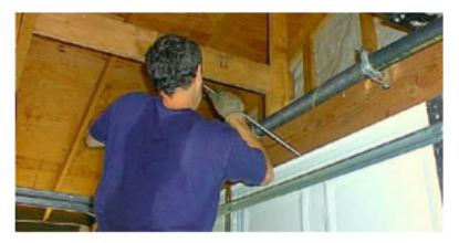
It is important to check the tension of the~ springs. Disregard the electric door opener, if you have one, and try to open the door manually.
